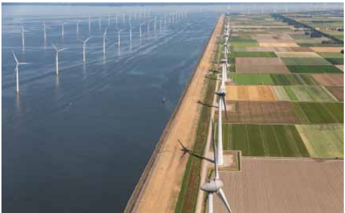
Aerial view Dutch landscape with offshore wind turbines along coast. © T.w. Van Urk | Dreamstime.com
